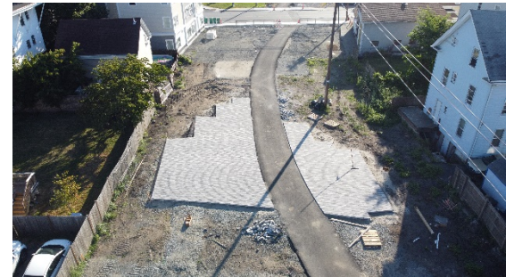
Concrete pavers installed throughout Linear Park
