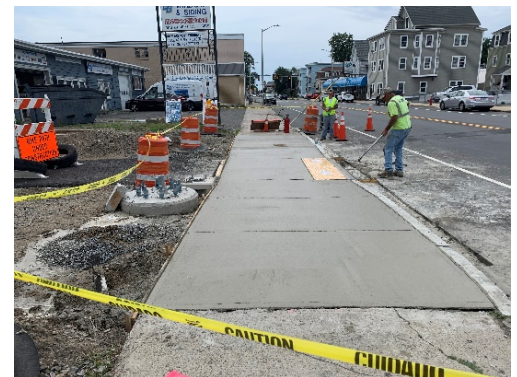
Install new granite curbing and pour concrete sidewalks from Summer St (2) through Boston St
