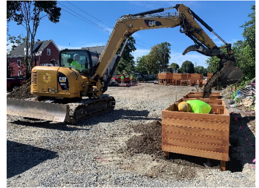
Begin installation of community planters in Linear Park
