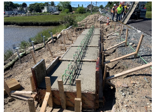
Placed concrete for Lynn overlook
