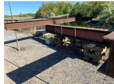
Testing Helical pile at Bridge 1 east abutment
