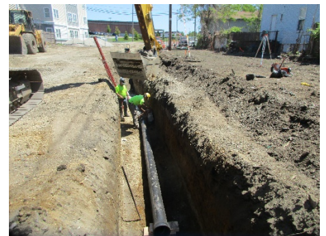
Linear park irrigation system in progress
