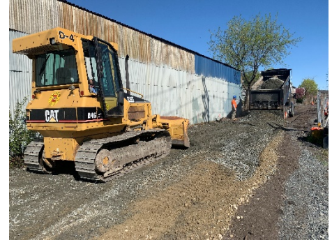
Gravel for subgrade from Project End through Summer St (2)
