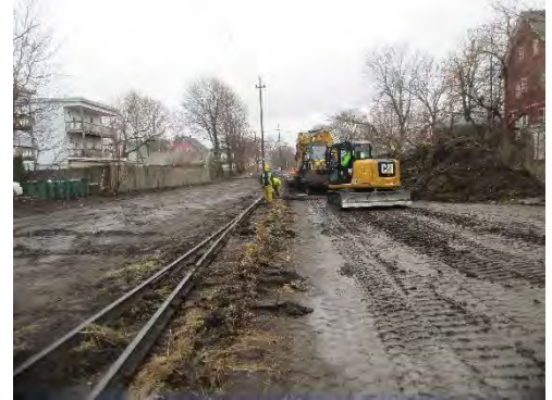
Rail removal through Linear Park
