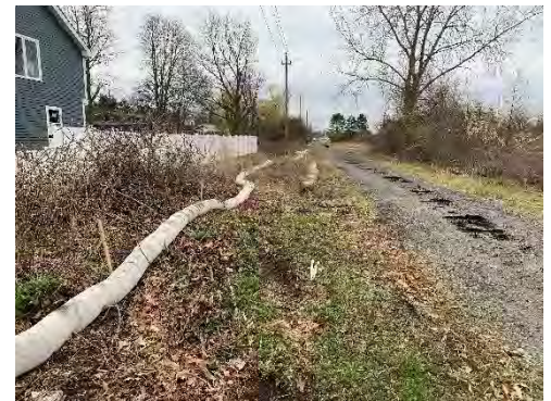
Erosion Control placed from Central St through Boston St
