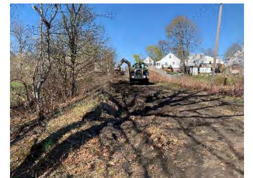
Track Excavation and clearing/cleaning from Ashland St through Cottage St.
