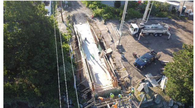
Placed concrete for Bridge 1 east footings, abutment, and wing walls
