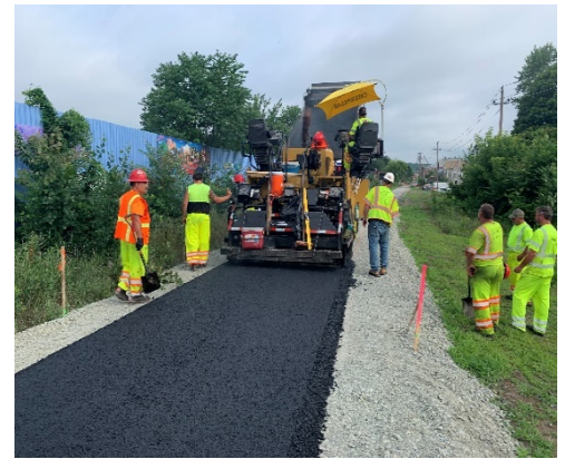
Pave trail with intermediate course from Bennet St Bridge through Boston St (401+50 to 486+30)
