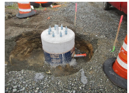
Western Ave mast arm foundation installed
