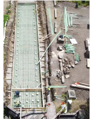
Helical piles installed, cut, and capped at Bridge 1 east & west abutment/footing
