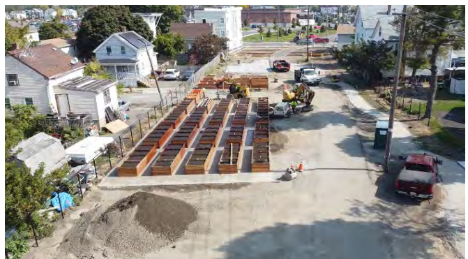
Overview Linear Park Community planter installation progress
