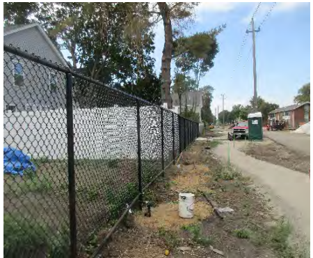
Fence Installation Linear Park in Lynn South side
