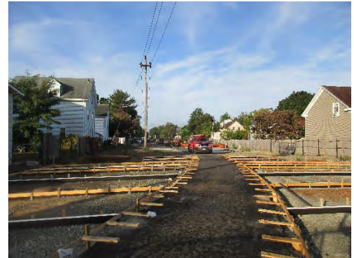
Forming for concrete food truck plaza in Linear Park in Lynn
