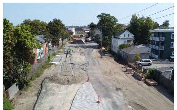
Overview Linear Park Playscape installation progress
