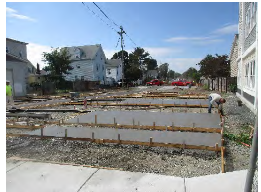
Start of concrete placement Linear Park food truck plaza
