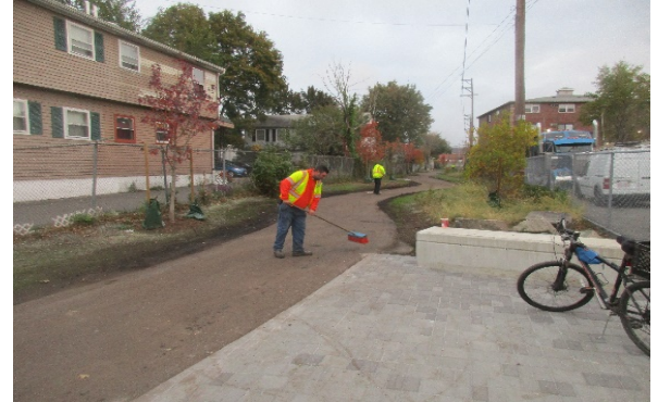
Preparation for Placing Pavement Sta. 472+50
