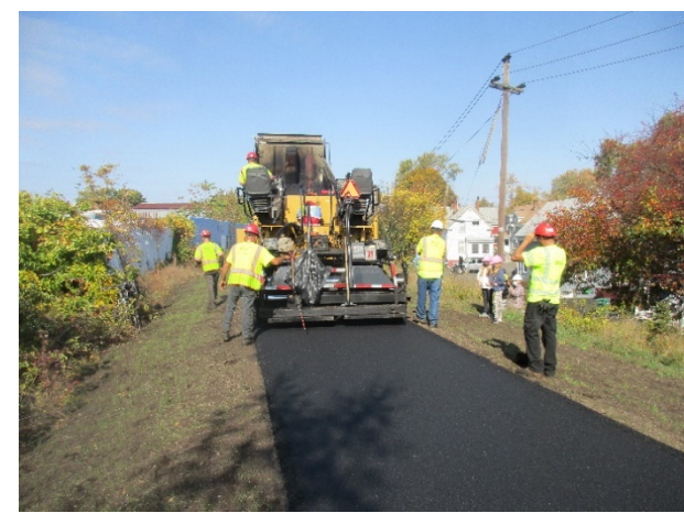
Top Course Pavement Sta.482+00
