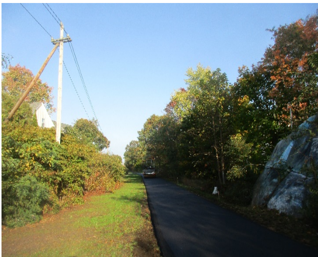
Pavement along trail Sta. 435+50
