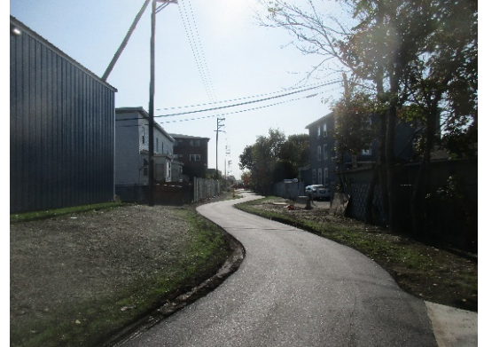
Top Couse Pavement Sta. 467+00
