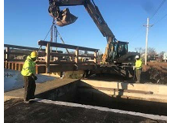
Hoisting and placement of Bridge 2
