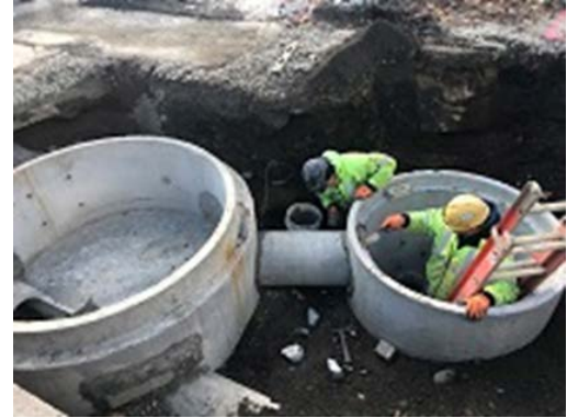
Denver St drain manhole and catch basin installation (STA 257+00)
