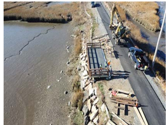
Progress of Lynn overlook
