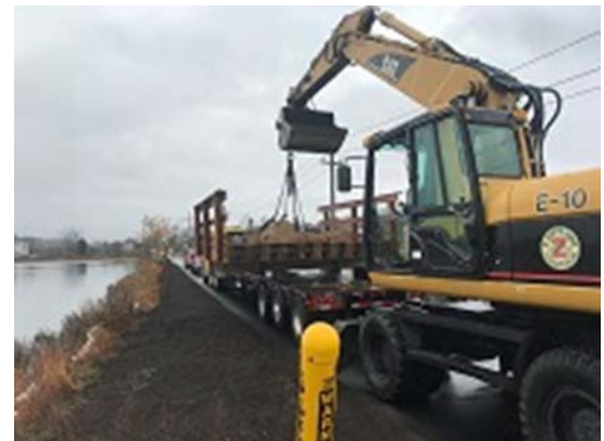
Hoisting and placement of Bridge 3
