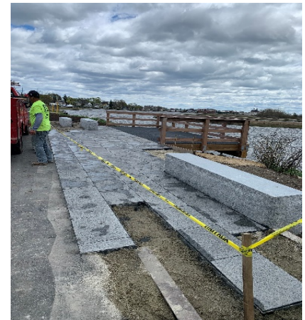
KDC installing Granite Paving & Benches @ Lynn Overlook
