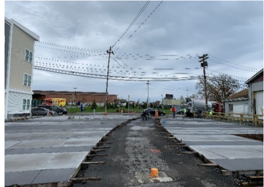
KDC Pouring Concrete (4000 psi) for Colored Cement Concrete Plaza @ Linear Park.
