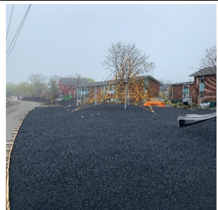
FIBAR PIP Rubberized base safety Surfacing installation at Linear Park.
