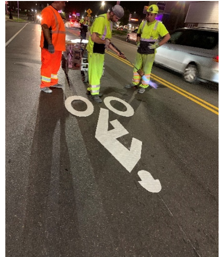
Road Safe installing pavement legend BIKE at Western Ave. Lynn.
