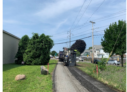
Garrity Asphalt Reclaiming Inc. Milling existing bike path Malden/Revere path line
