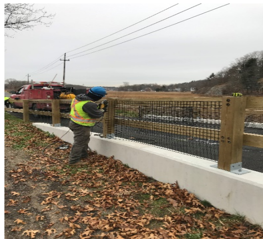
RZC installing Wire Mesh for Bridge 1 approaches at Saugus.
