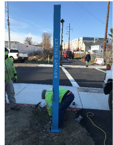
RZC installing Street Signs at Bryant Street, Malden.
