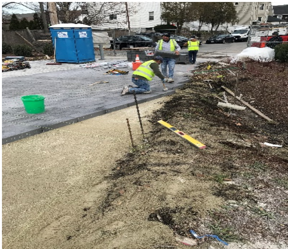
K Da Ponte installing pre-cast concrete pavers at West Street, Everett.
