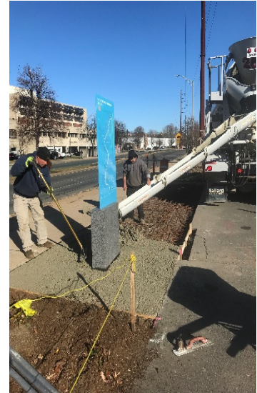
RZC installing Concrete Pad at Ferry Street, Malden.
